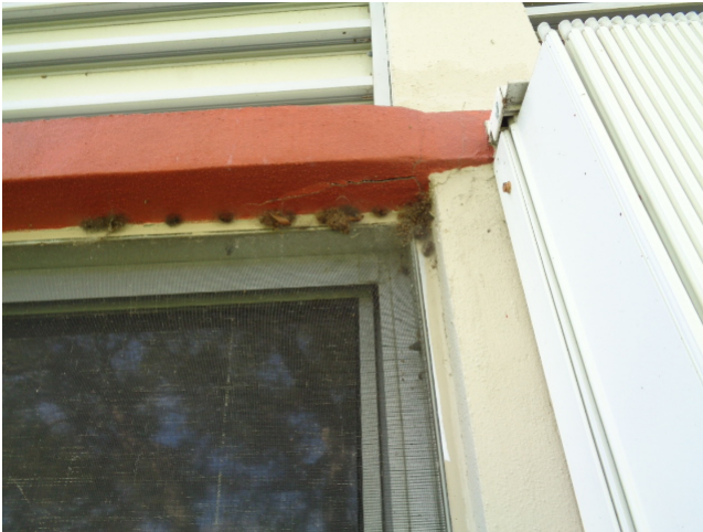
Figure 12...Edge spalling
