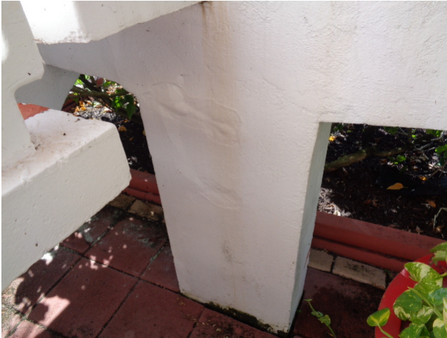
Figure 7...Column spalling at east stair
