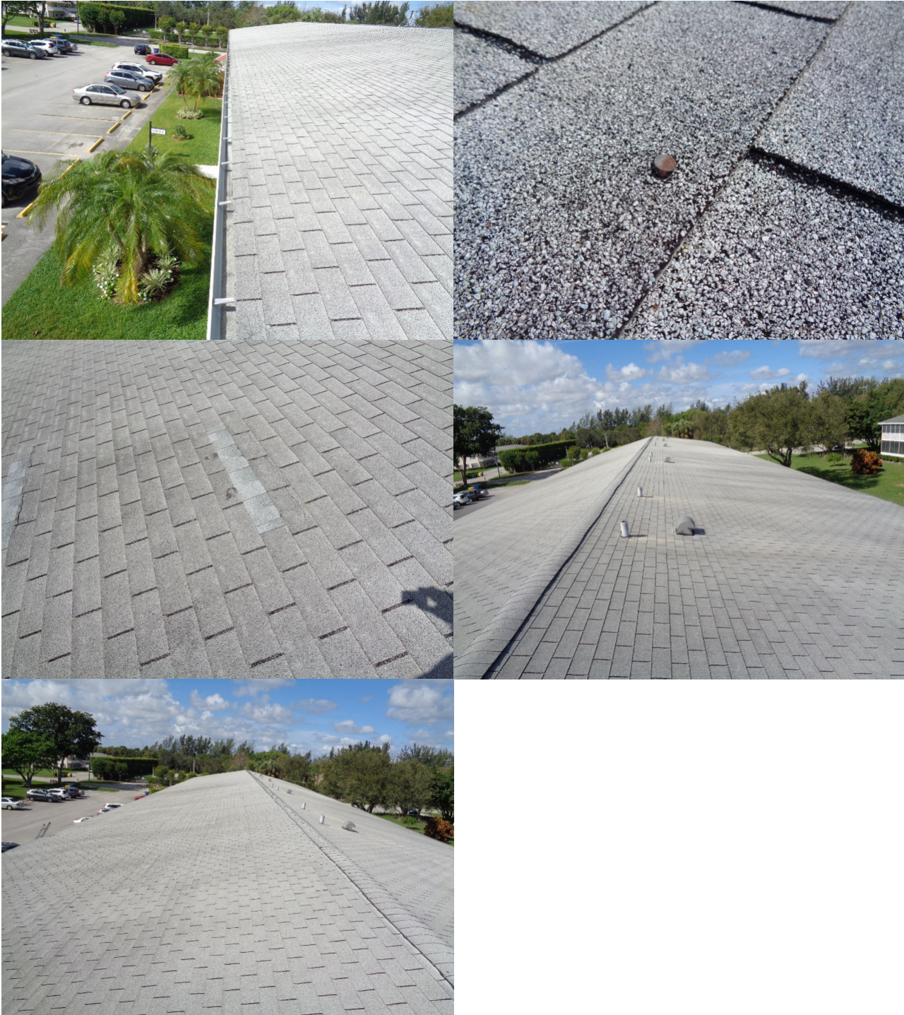
Figure 6...ROOF Pictures show repairs and backed out nails
