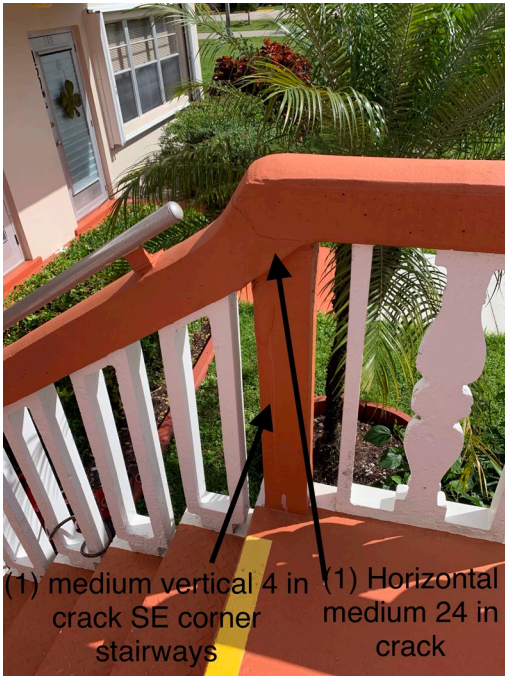
NCI-9: Cracked concrete SE stairway post
