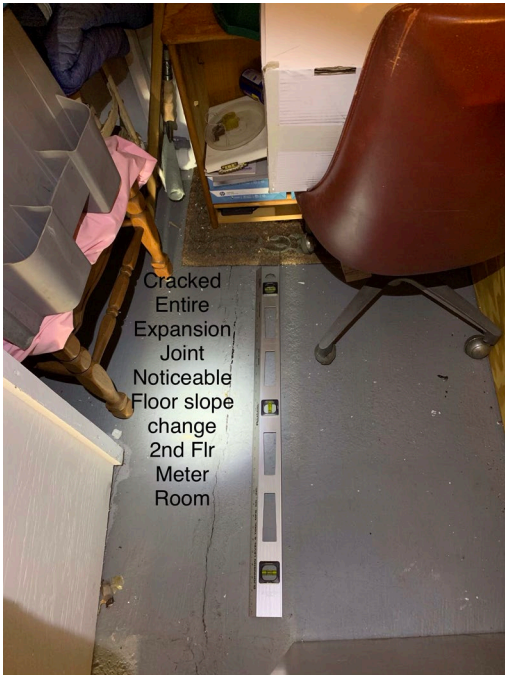
NCI-10: Cracked entire expansion joint and change of floor slope
